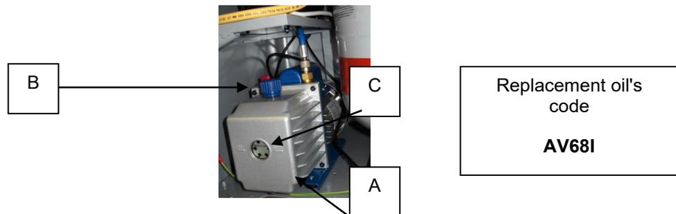
Image 51 - The pump and its elements
